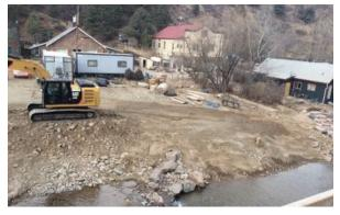
**GOAL:** to restore the Town Square to its pre-flood elevation – includes debris removal, excavation & creating new contour lines, importation of fill and top soil.
