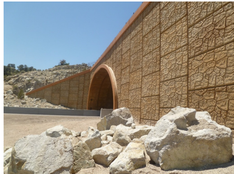
Concrete Panel MSE Wall Examples
