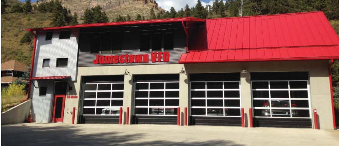
Figure 7-4: Jamestown Volunteer Fire Department Fire Station
