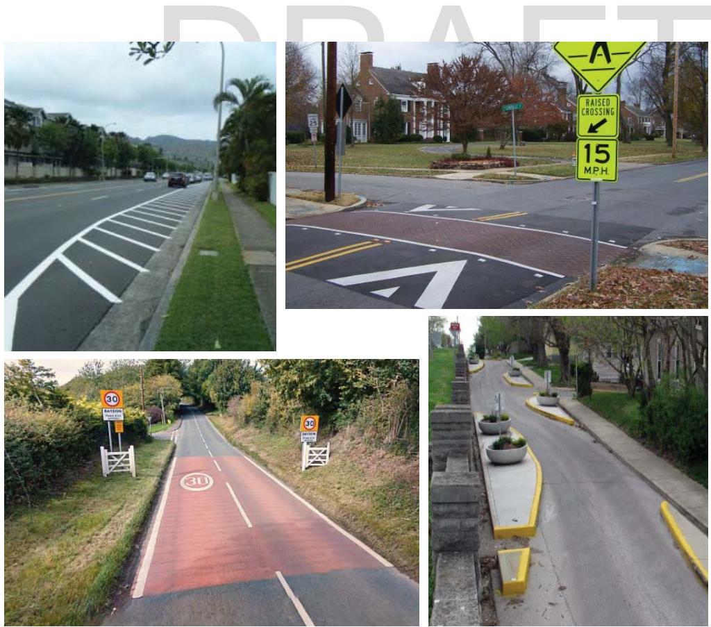
Figure 5-5: Example approaches to traffic calming that may be considered along Main Street / County Road 94 - striping (upper left), raised crosswalks (upper right), signage and paint / pavers (lower left), bump-outs (lower right)
