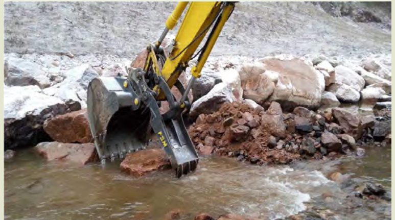
Excavator installing rock vane.
