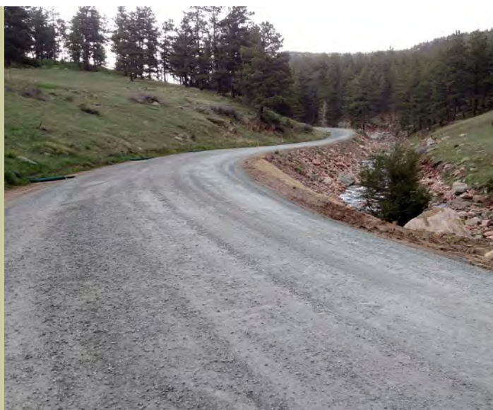
Geer Canyon Drive now has a completed road and a new completed set of culverts as of this spring.
