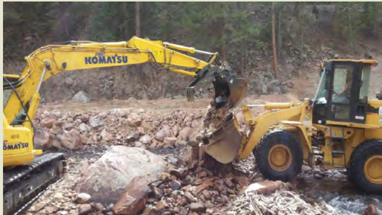
Excavating a low flow channel on the North St. Vrain Creek.
