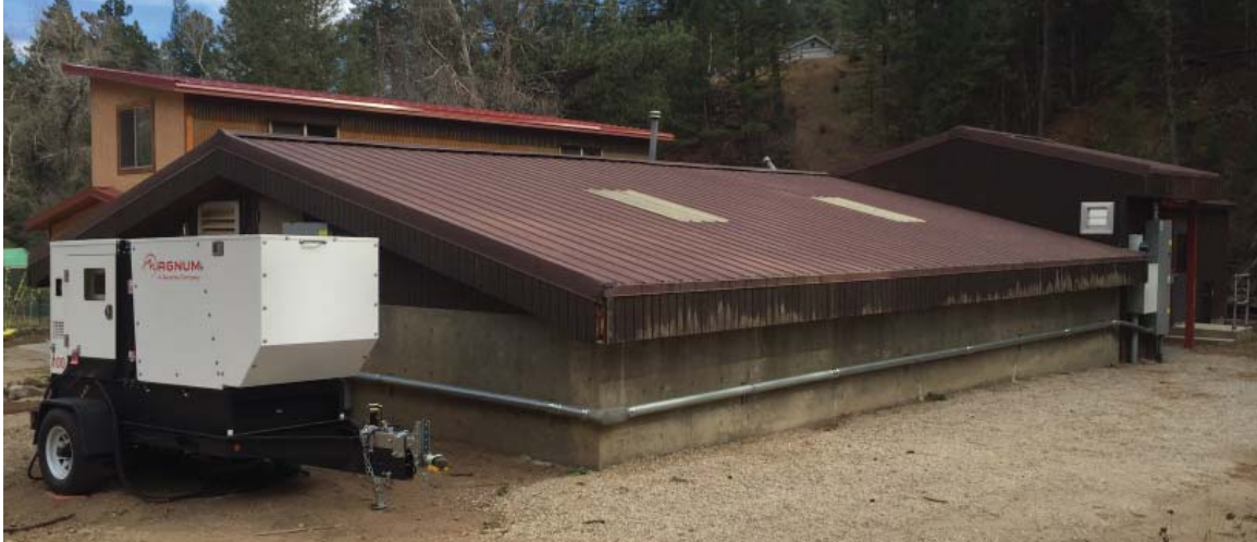
Figure 6-2: Jamestown Water Treatment Plant
