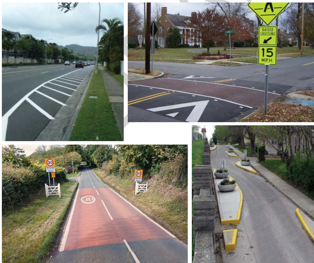
Figure 5-5: Example approaches to traffic calming that may be considered along Main Street / County Road 94 - striping (upper left), raised crosswalks (upper right), signage and paint / pavers (lower left), bump-outs (lower right)
