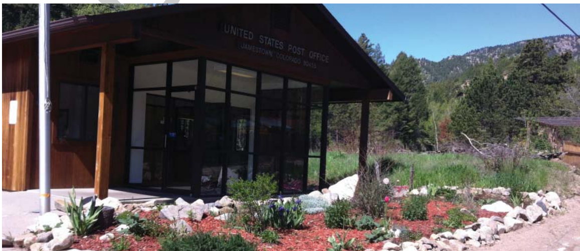
Figure 7-4: Jamestown Post Office
